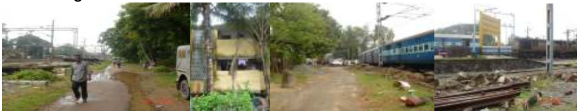
Figure 5.6.36: Site Conditions- Ernakulam Junction Station
