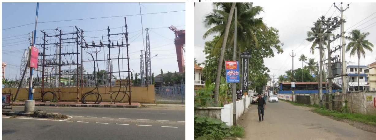
Figure -6: Overhead electrical and telecommunication cables with poles and substations on footpaths
