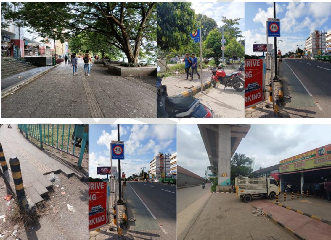
Figure 44 Condition of Footpaths & NMT Facilities (Source: Primary Site Visits-2022)
