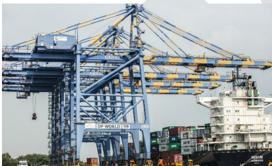
International Container Transshipment Terminal
