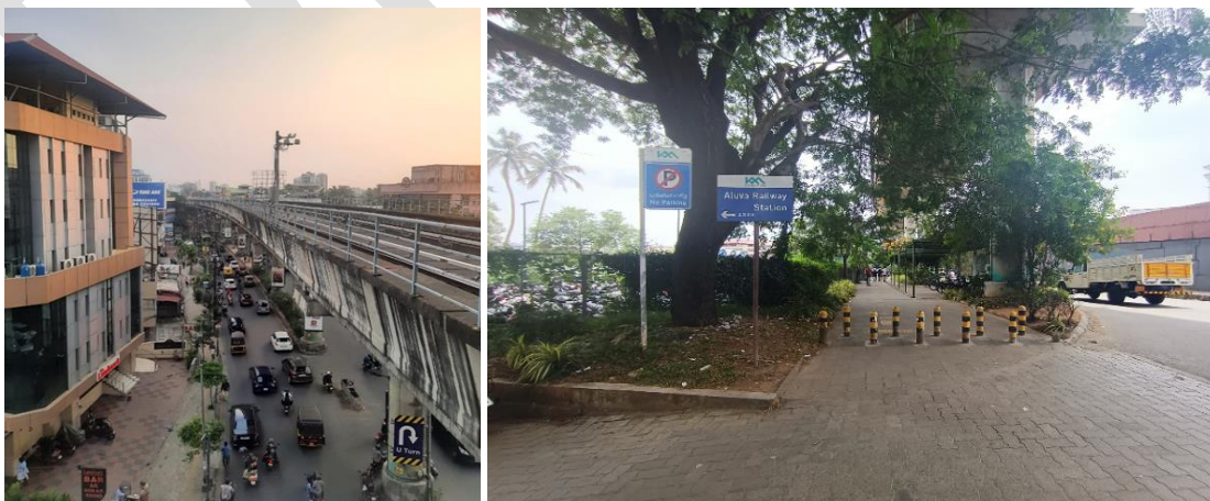
Figure 78 Dedicated Pedestrian Facilities provided along Banerji Road and NH 544 (Near Aluva)
