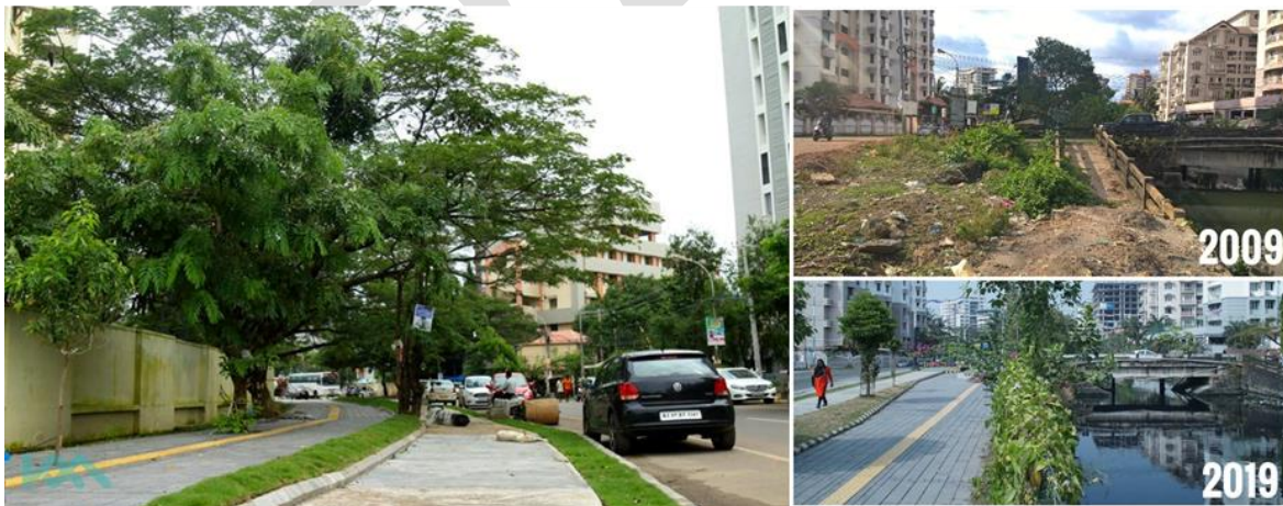
Figure 157 NMT Shihab Thangal Road, Panampally Nagar, Kochi as a Pilot Project by KMRL (Source: KMRL, Twitter)
