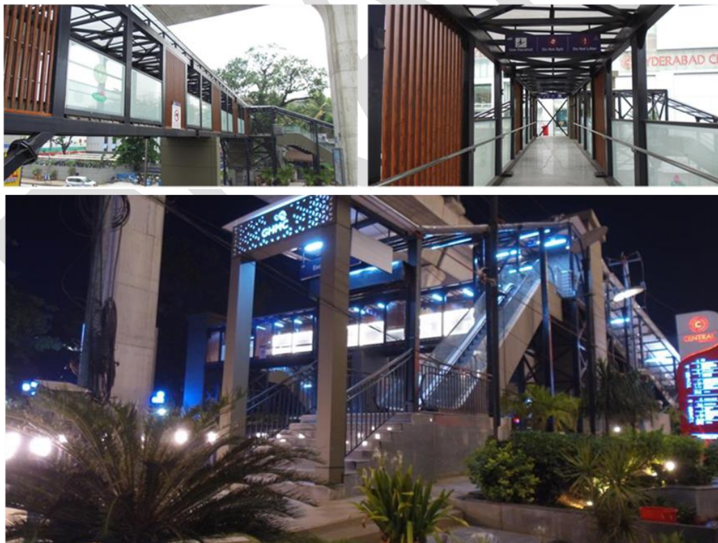
Figure 182 FOB at Punjagutta Central with Escalators, Lifts and Stairs, Hyderabad
