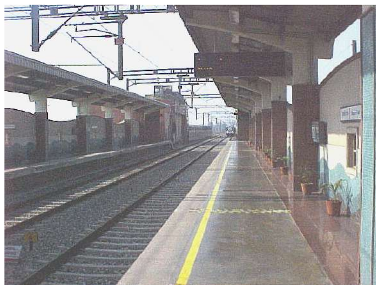
Typical 25kV AC Catenary Arrangement
