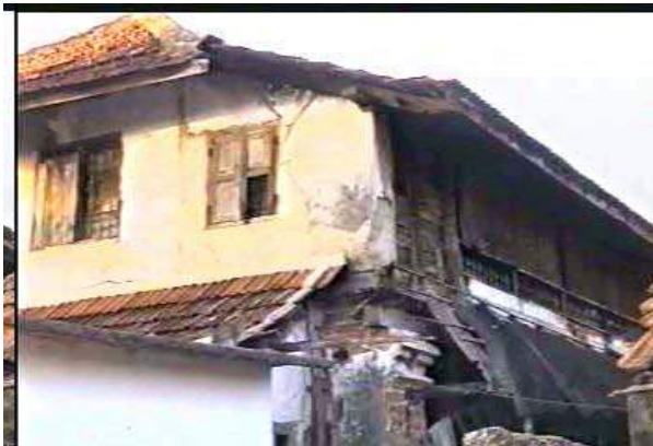
Figure 7.5: A Rehabilitation Project under DFID
