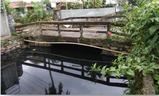
Ch 8200 Foot bridge construction reducing water way in Chilavanoor
