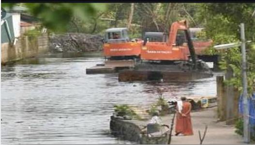
**Figure 4A.3(a) Hitachi fixed on a pontoon for deepening**
