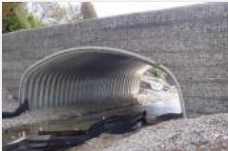
**Figure 4A.19: Head wall protection (Rock face wire mesh with MSE)**
