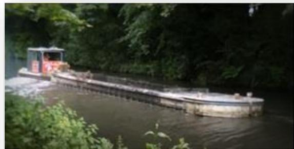
**Figure 4A.3(d) Excavated material conveyed by barge for disposal**
