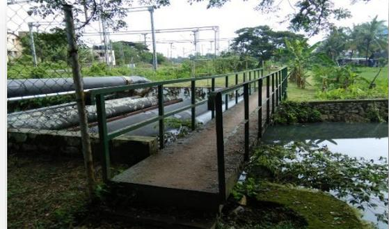
Ch7330 Lack of vertical clearance of foot bridge and utility crossing at Chilavanoor canal
