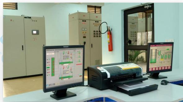
**Figure 4B.12: SCADA lay out for a Sewage treatment plant**
