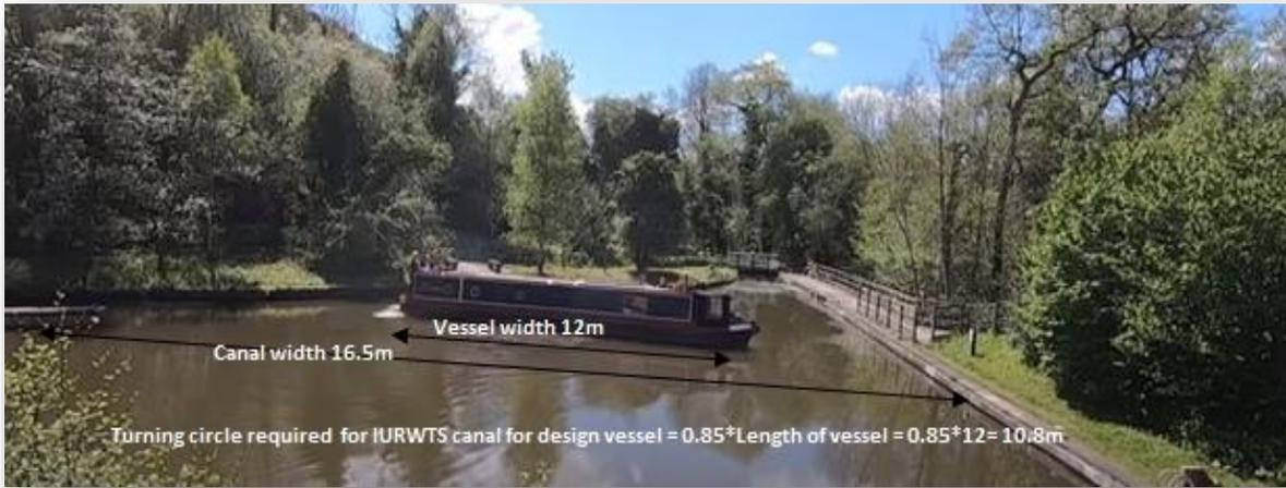
*Turning circle: Vessel In the process of turning in the canal*
