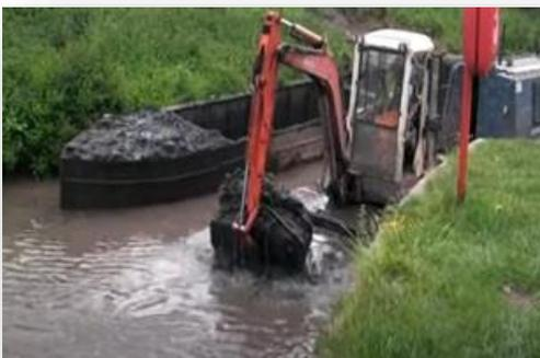
**Figure 4A.3(e) Machinery for deepening smaller canals**
