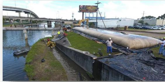
**Figure 4A.3(h) The sucked earth from Dino 6 dredging used to fill geo-synthetic tubes**
