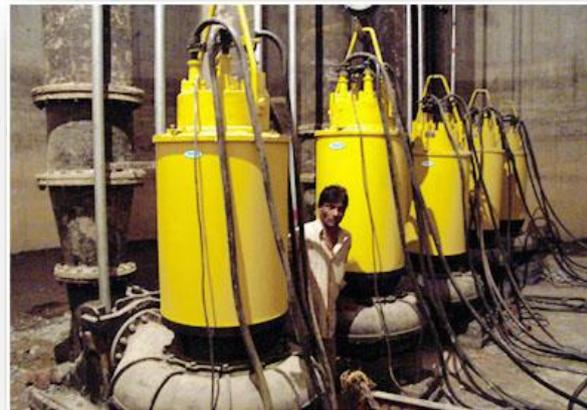
**Figure 4B.3: Intermediate pumping systems**
