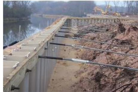
**Figure 3A.27: Typical anchored sheet pile**
