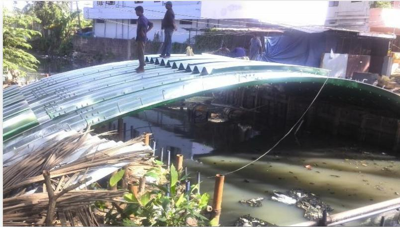
**Figure 4A.21: Construction of CSP arch bridge across T-P canal at Kochi**
