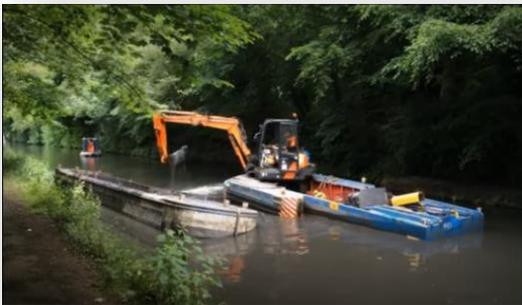
**Figure 4A.3(c) Excavated material filled into barge**
