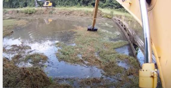
**Figure 4A.3 (b) Long arm deepening Hitachi**
