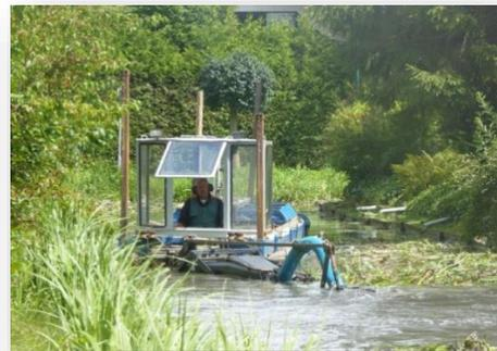
**Figure 16.6: Debris removal using mechanized vessels and canal mowing**
