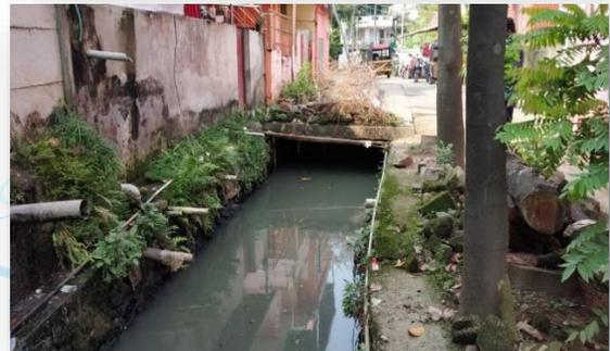
Ch 3460m Chilavanoor canal vent way reduced and covered by slabs to increase road width
