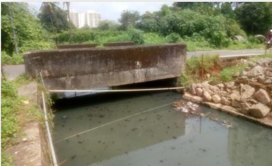
Ch 5570 Chilavanoor canal vertical clearance less than a metre
