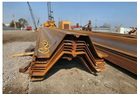
**Figure 3A.29: Cross sectional view of steel sheet pile**
