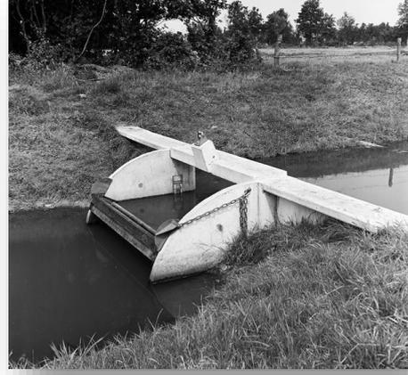
**Figure 16.8: Examples of spillway and closing locks**
