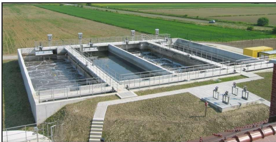
Figure 11: Photo image of SBR technology plant
